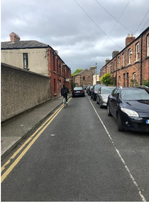
Figure 8: View from Cork St. access towards Development on Rehoboth Place
