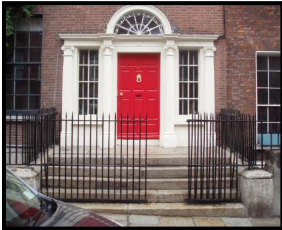
Figure 48 – No. 41 North Great Georges Street entrance doorway with sidelights, fanlight & iron gates
