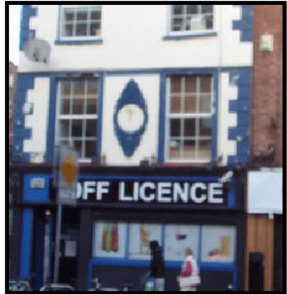
Figure 52 - Decorative stucco panel and quins at corner of Parnell Street & North Great George's Street
