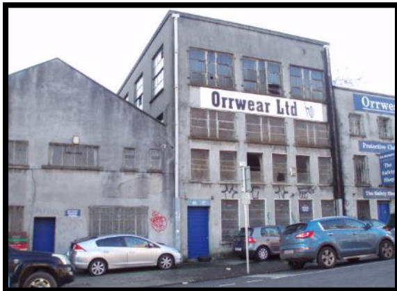
Figure 21 - No's 40-42 Hill Street – 20th Century light industrial and warehouse building character
