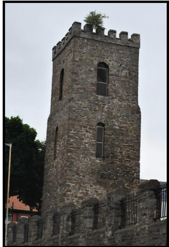
Figure 23 – St. George's Tower, Hill Street
