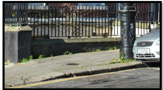
Figure 58 - No. 20-21 North Great Georges St - Original granite paving contributes to the appearance of the 18th Century streetscape
