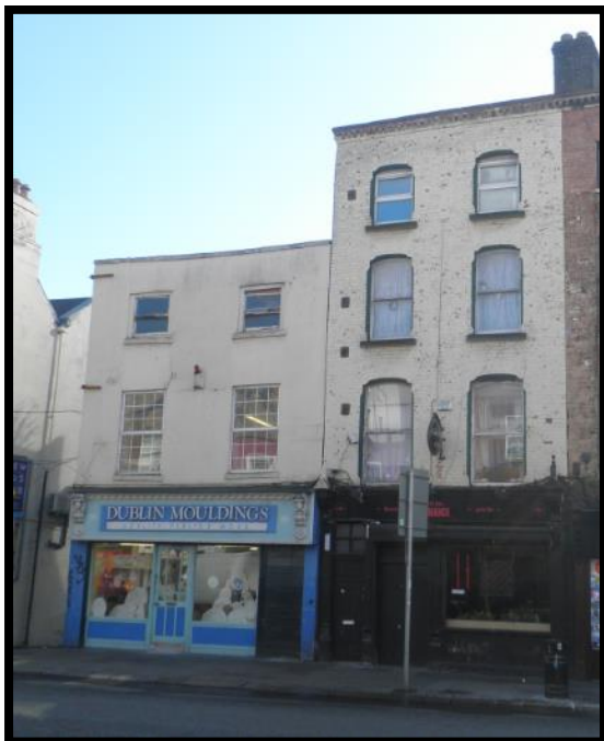
Figure 36 – No's 98-99 Parnell Street earlier 18 th Century structures refaced in the 19 th Century
