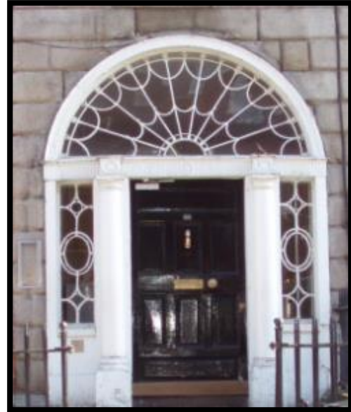
Figure 46 - No 46 North Great Georges Street – elaborate fanlight and sidelights to 18th Century townhouse
