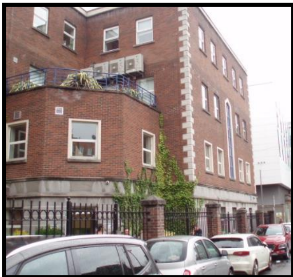
Figure 33 - Four storey structure onto mews lane Nerney's Court
