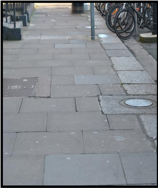
Figure 59 – Gardiner Place - Mix of replacement concrete paviors, tarmacadam infilling and historic granite kerbs
