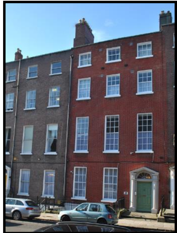
Figure 25 - Late 18th Century terraced buildings – no's 7-8 North Great George's Street
