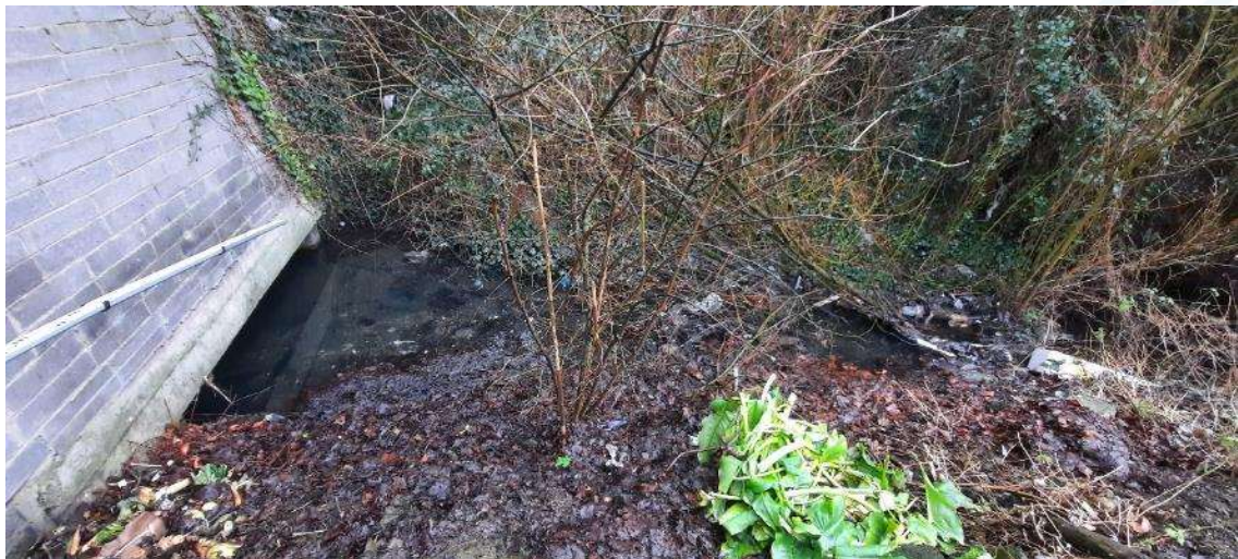
Figure 2-5 Finglas Stream Open Channel Section (Facing East)
