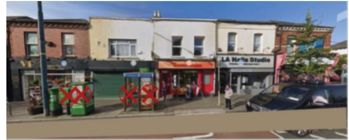
Figure 6.5. Berkeley Road. Street clutter could be removed (red crosses) and the street could be widened (beige strip). This would allow for fewer obstacles for pedestrians, while also allowing for outdoor seating for business.
