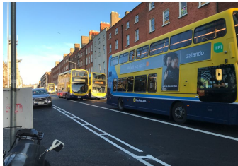
Condition of Existing Route
